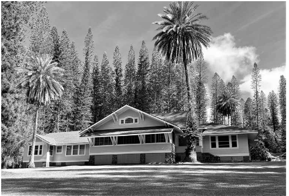
Formerly the plantation manager's residence (1920s), the Social Hall is now used as lodging for off-island visitors, construction workers or visiting relatives for family reunions. Photography by Nel Cabiles
